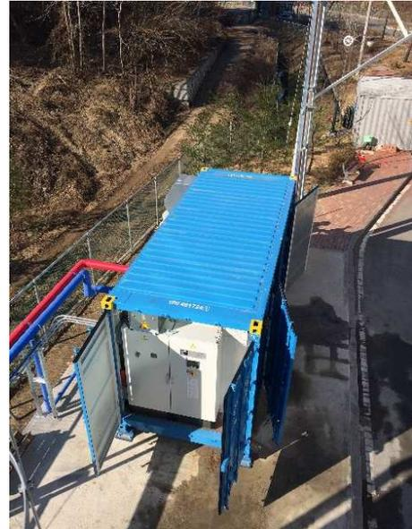
On average the ORC machine consumes 1.5 tonnes/hour of steam at 143°C which is condensed and subcooled to 80°C by the E-RATIONAL HT-ORC, recovering 1000kW of heat. Under these conditions, the machine is operating at part load capacity. At full load capacity (of 1500kW of heat) the machine is producing around 135kWe.
