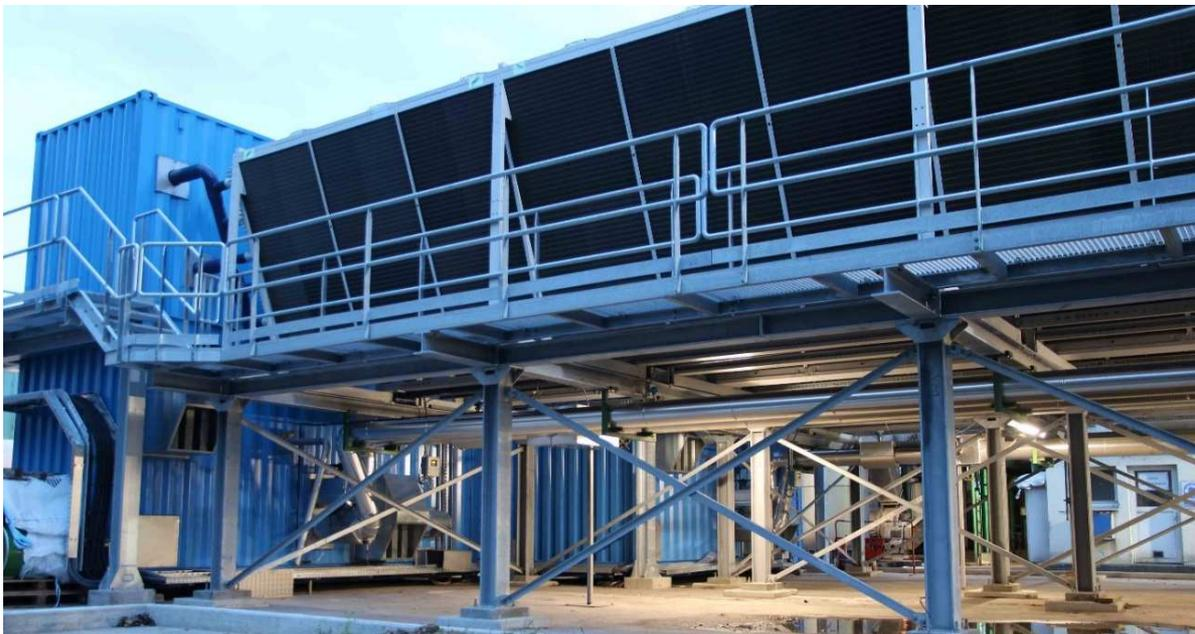
*Unit 2 – E-RATIONAL ORC 20FT – 3MWTH – 370KWE with direct air cooled condensers*
