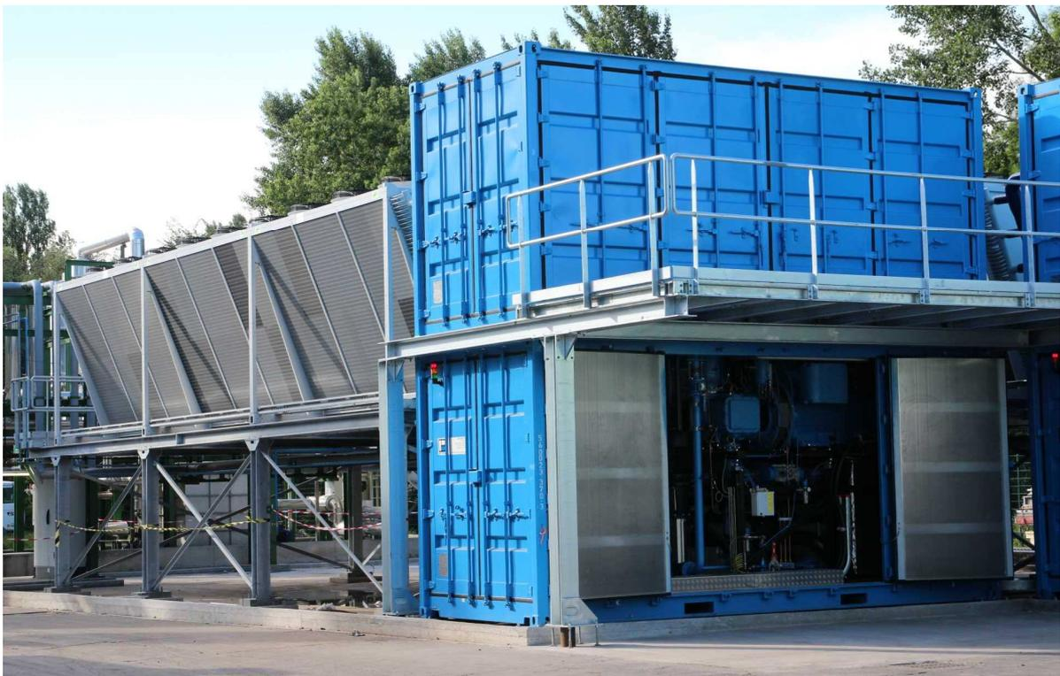
*Unit 1 – E-RATIONAL ORC 20FT – 3MW<sub>TH</sub> – 370kWe with direct air cooled condensers*
